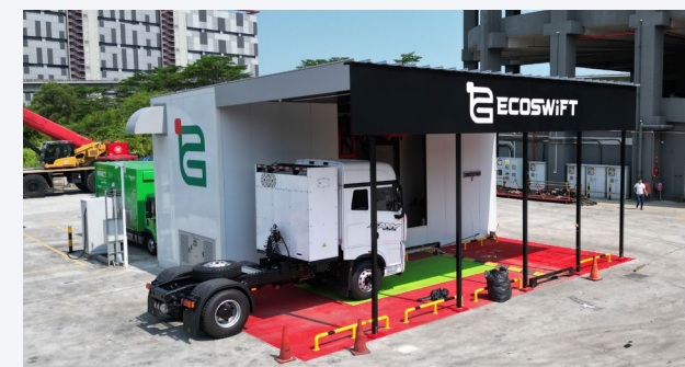
Launch of ECOSWIFT's battery charge and swap station in Tuas, Singapore – the country's first public facility for electric heavy commercial vehicles on 1 August 2025.
